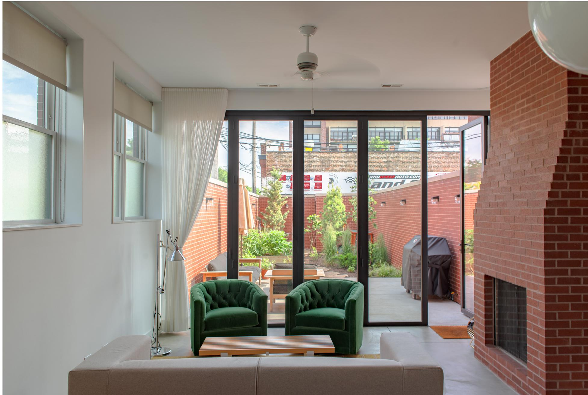
The doors are triple paned and filled with Low E Argon gas to protect against the cold Chicago winters while still allowing sunlight to fill the rooms from floor to ceiling.
