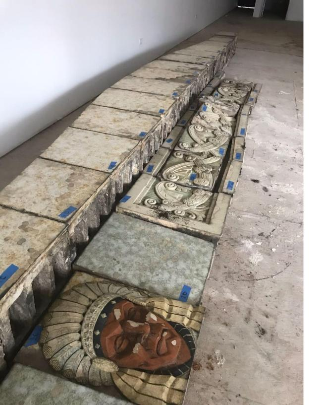
As each piece came off, they were kept onsite. The facade was reassembled, this time the floor, inside the building. This allowed the team to clearly see the pieces up close and inspect every side of them. Finally, a full picture of the facade's overall condition could be thoroughly visualized.
