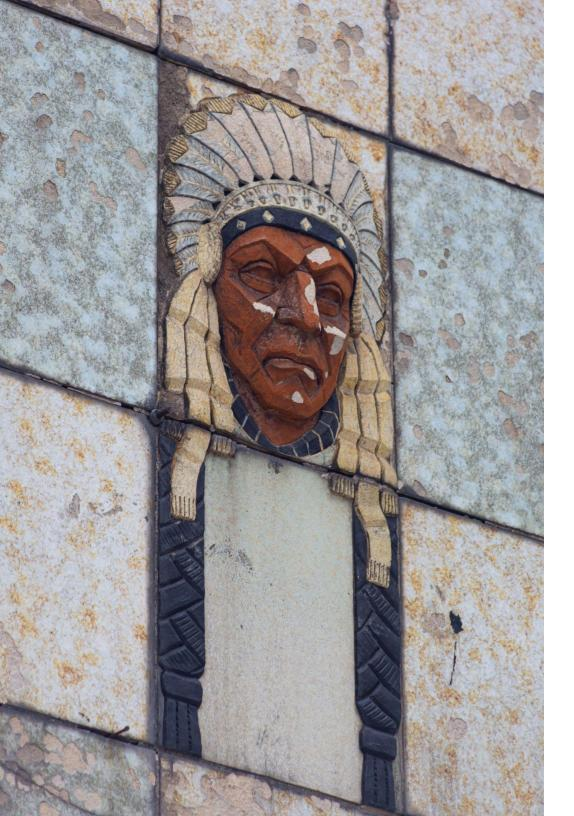
Unfortunately, the faces had not fared any better than the blocks. They were left chipped and broken; hardly recognizable from their state during installation nearly 100 years earlier. The face shown on the right was covered in so much soot and dirt, that all the angular demarcations had nearly been lost. On the left, the face had lost large pieces of the cheek, chin, nose and forehead. On both, feathers on the headdresses had were mostly lost.
