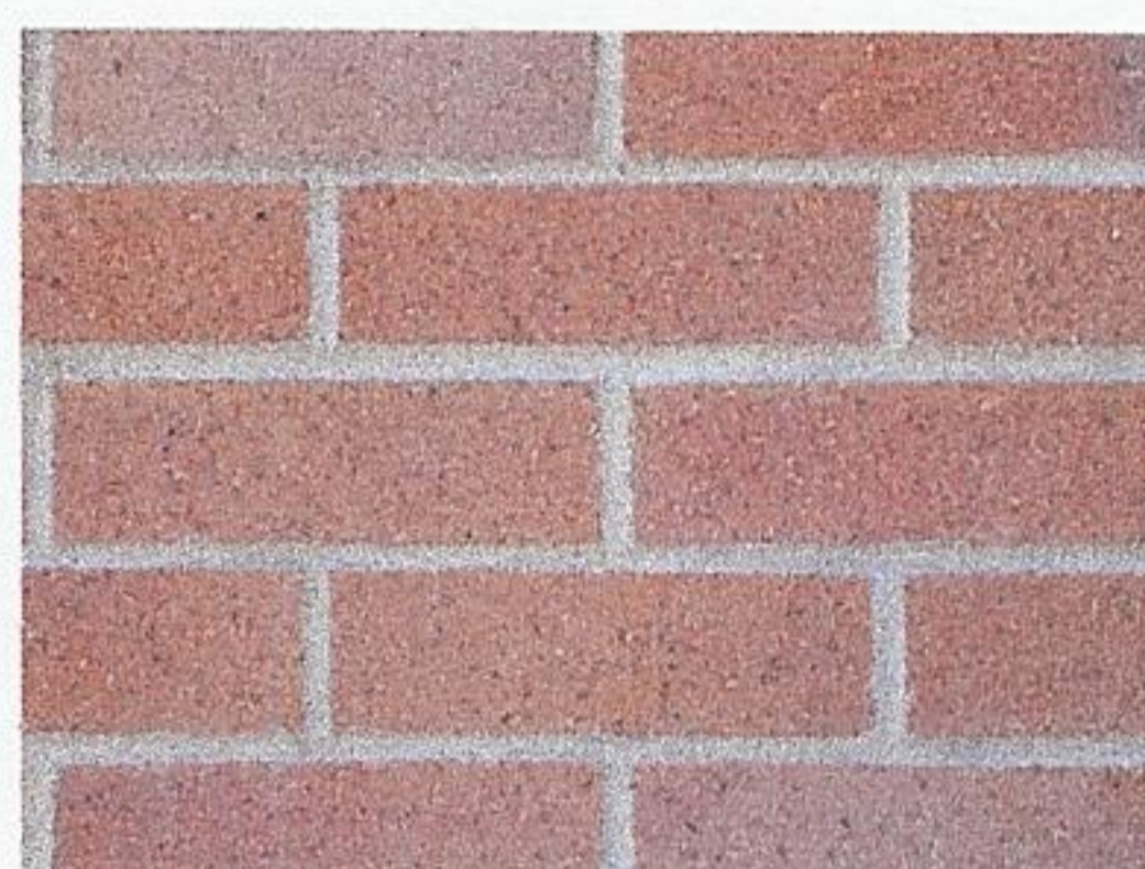
50/50 SLOTTED 16" BRICK AT TWIN GROVE ELEMENTARY, BUFFALO GROVE, IL
