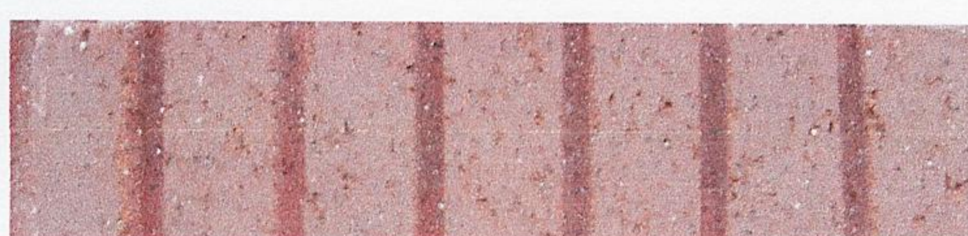
This is a 16" thru wall brick with 7 slots! (Wheeling Animal Hospital, Wheeling, IL)
