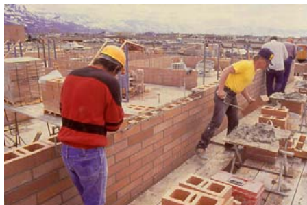
Mason contractors laying 8"x4"x16" structural thru wall brick
