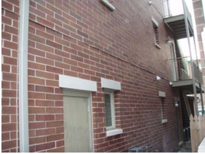
Thru-wall brick at Park Blvd (35th and Federal), Chicago IL.
