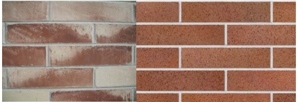
The aesthetic differences between clay and cement can be seen in these two photos
